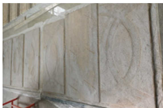
9. Leveling the pattern by net and sand
