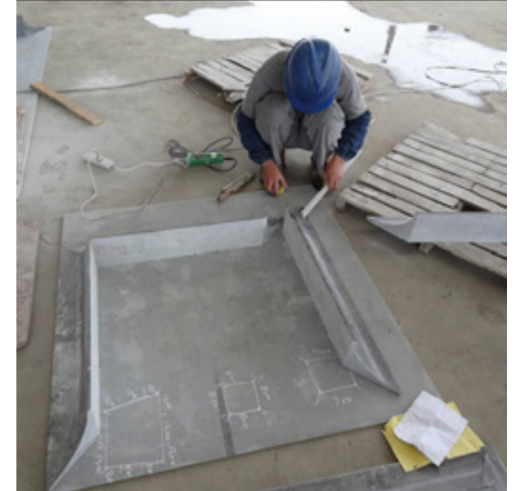
4. Process of jointing
